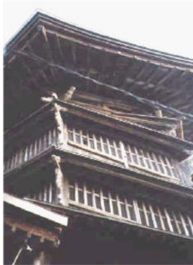
(3) Photograph of the tower showing helical structure
